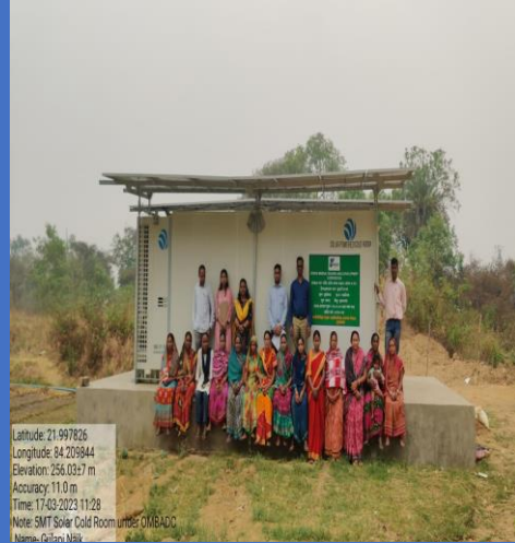
5MT SOLAR COLD ROOM(OMBADC) SADAR SUNDARGARH
